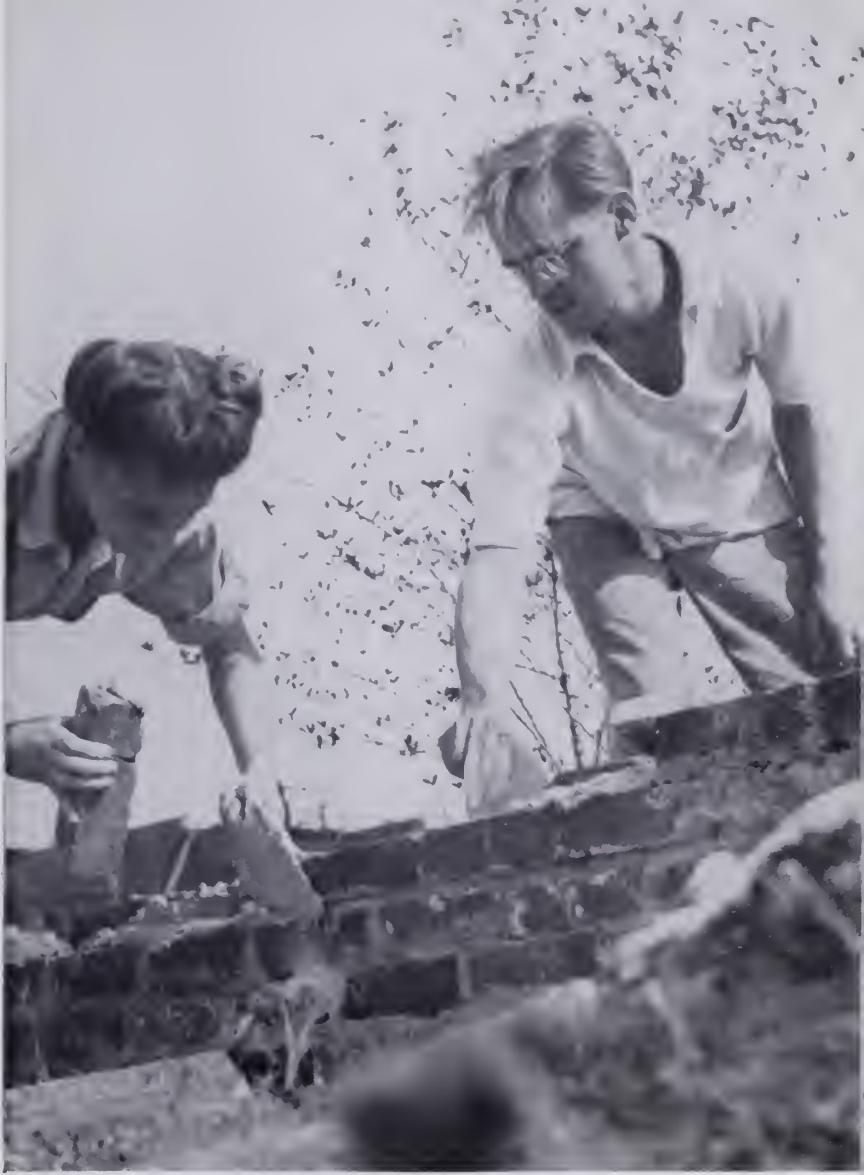
Work campers and members of the local community worked together to build Flanner House, Negro Community center in Indianapolis, Indiana
